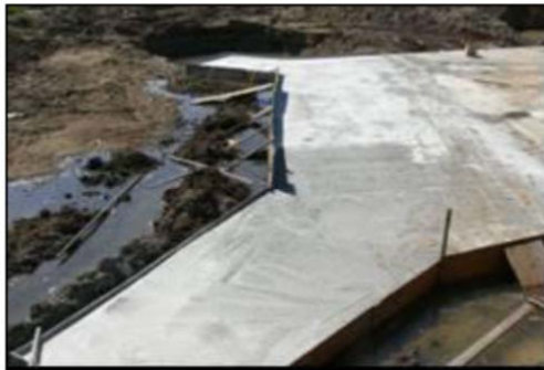
Construction of Low Level Stream Crossing and Haul Roads
