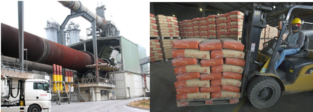
Cement Manufacturing Plant & Cement Product Storage
