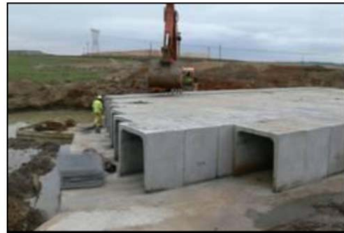
Construction of Low Level Stream Crossing and Haul Roads
