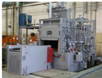
Installation of Ipsen Furnace
