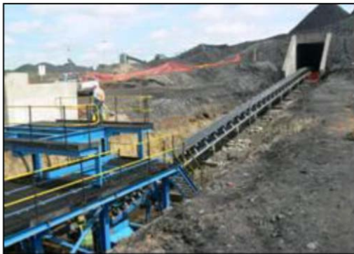
Construction of Conveyor and Feeder Breaker
